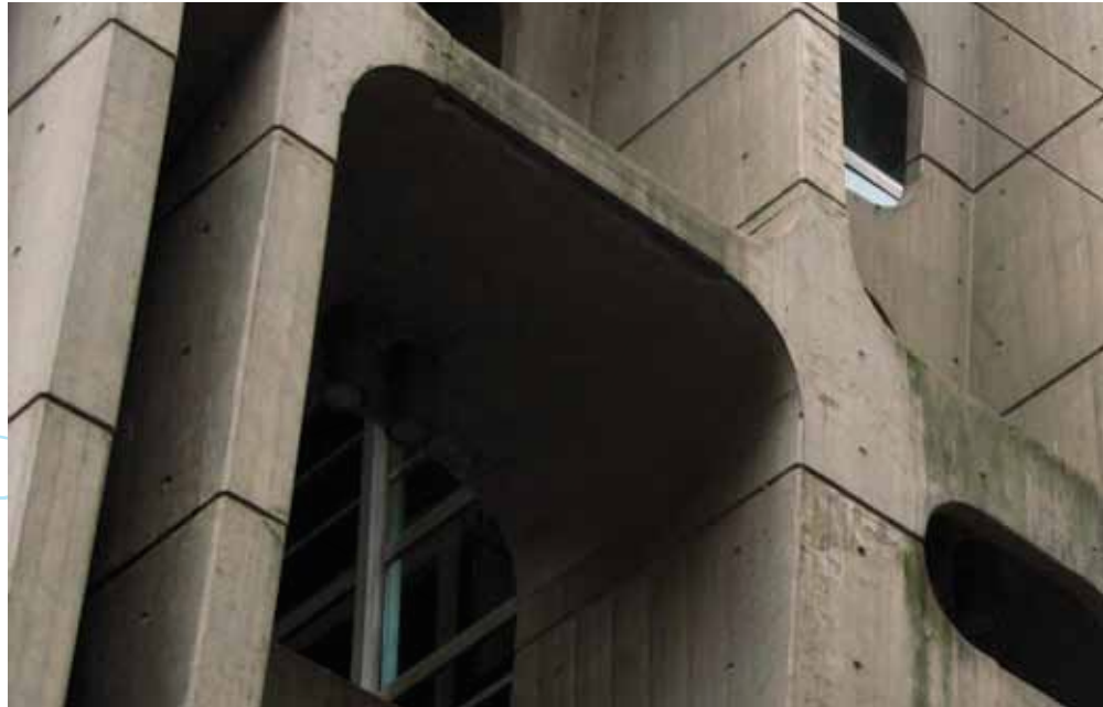
The Bank of London (now 'Banco Hipotecario') by Clorindo Testa Argentine architect
