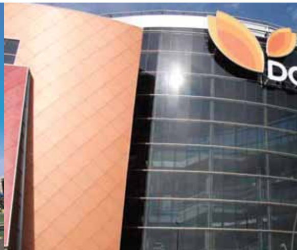
DOT Baires Shopping in Buenos Aires, Argentina, built by IRSA Group
